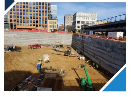
double insulating blankets and heat during the curing process. Temperature sensors were also installed to track the shotcrete temperatures. The sensors showed that we were able to keep temperatures around 50 degrees or higher, allowing the shotcrete to properly cure and develop its structural strength.
