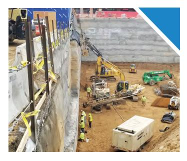
of alignment would have resulted in an additional construction cost of approximately \$250,000. To achieve the amount of verticality necessary, a customized mesh had to be fabricated rather than the typical flat mesh panels. The pre-stamped mesh was bent to fit behind the waler bars and anchor plates prior to applying the shotcrete.
